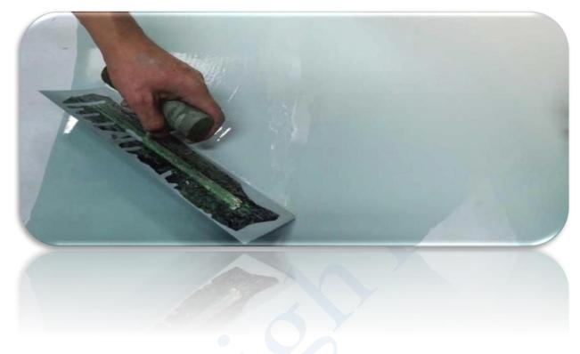
Hybrid polyurea is an elastomeric product of the reaction between an isocyanate and a mixture of composite resins, which due to its high penetrating power and adhesion is the best preparative and protection of concrete and metal substrates against moisture and corrosion. And it is a suitable primer before implementing the infrastructure of pigmented and protective coatings.
