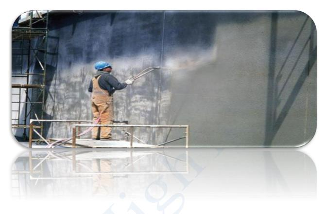
Powder Bluzed + is the most advanced type of crystalline waterproofing material with a high penetrating power into concrete capillary tubes, which is used to waterproof and protect concrete against the penetration of water and harmful chemical materials.
